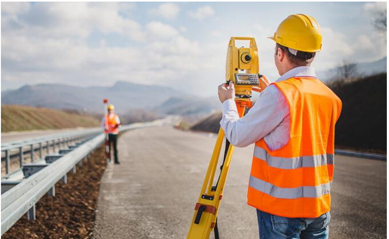
Fig. 1.Total station survey.
