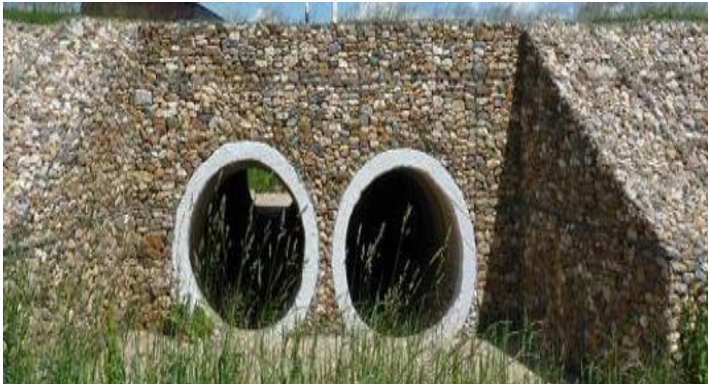
Figure-1. Reinforced concrete structures for water drainage.
