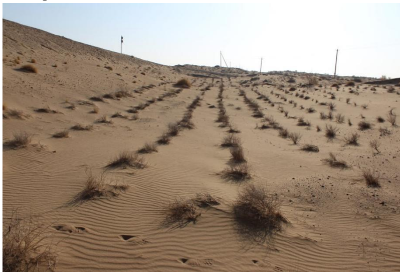
Fig. 1. Protection of the railway subgrade in sandy areas through grass seeding.
