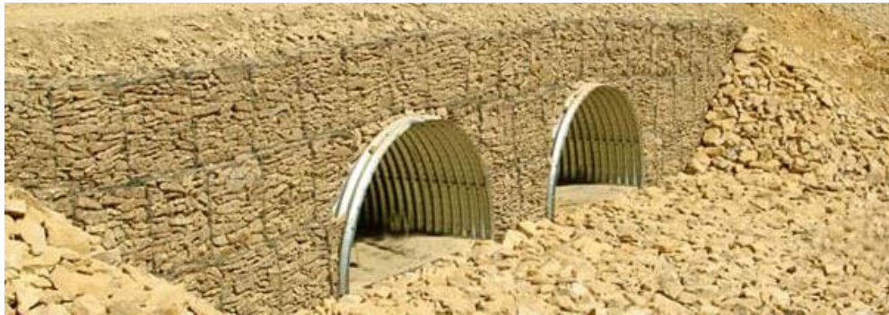
Figure-3. Culverts made of corrugated metal.
