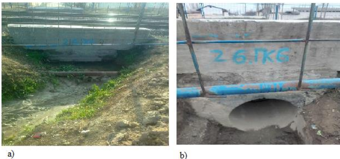
1-Figure. Condition of water pipes on the railway track
