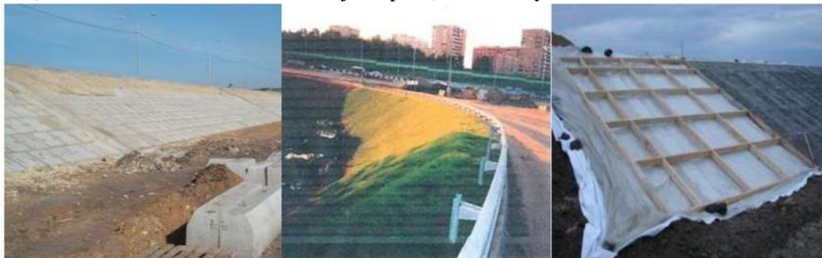
Fig.1. Protection of roadbed slopes
